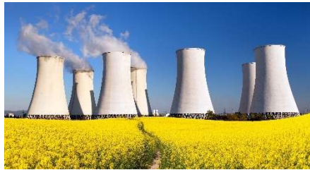
NUCLEAR POWER GENERATION
